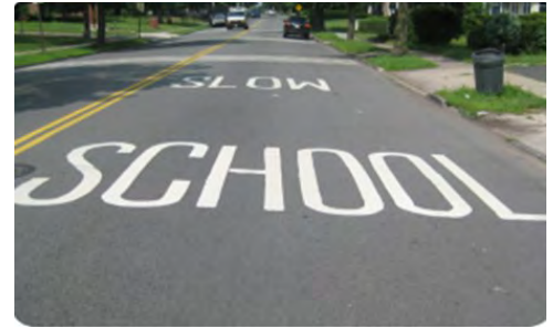
Slow school pavement markings.
