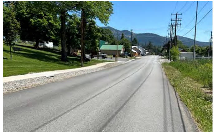
Existing High Street Sidewalk.
