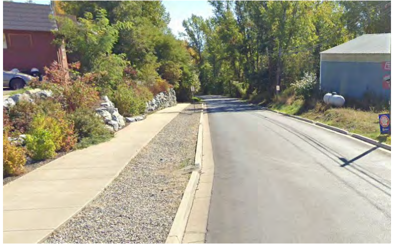
Existing High Street Sidewalk
