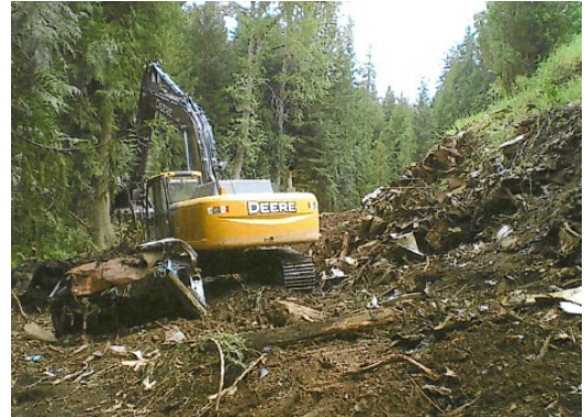
Figure 13: Former Priest River landfill site during remediation.
